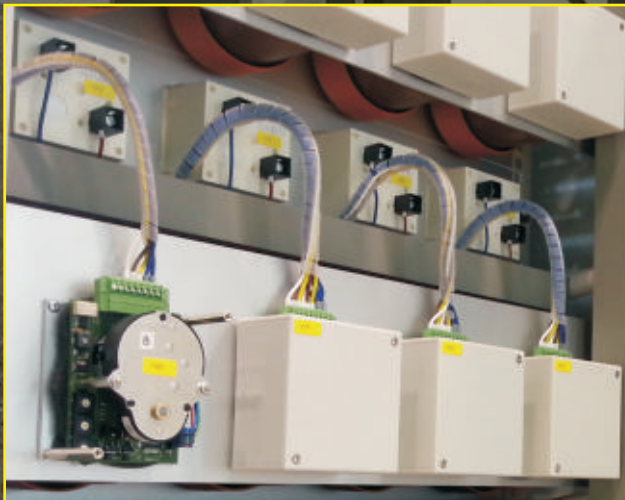
Example of retrofitting in LCP: Multi-channel protection device with remote control by stepmotor, all measurement and control channels on just one ISM2010 unit.
